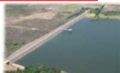
Presa Ing. Elías González
